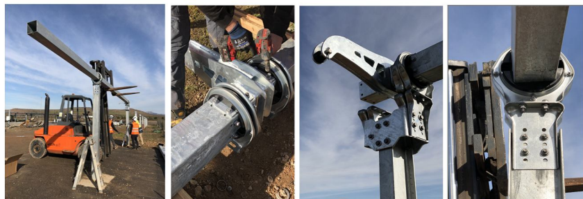
Assembly process of Torque-Tube and placement over the lower bearing supports
